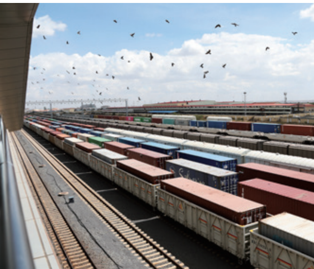
Freight trains at the Nairobi Station of the Chinese-built Mombasa-Nairobi Standard Gauge Railway in Kenya on November 17, 2021 (XINHUA)
