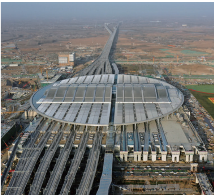
The Xiongan Railway Station of the Beijing-Xiongan intercity railway in Xiongan New Area, Hebei Province, on February 23, 2021 (XINHUA)
