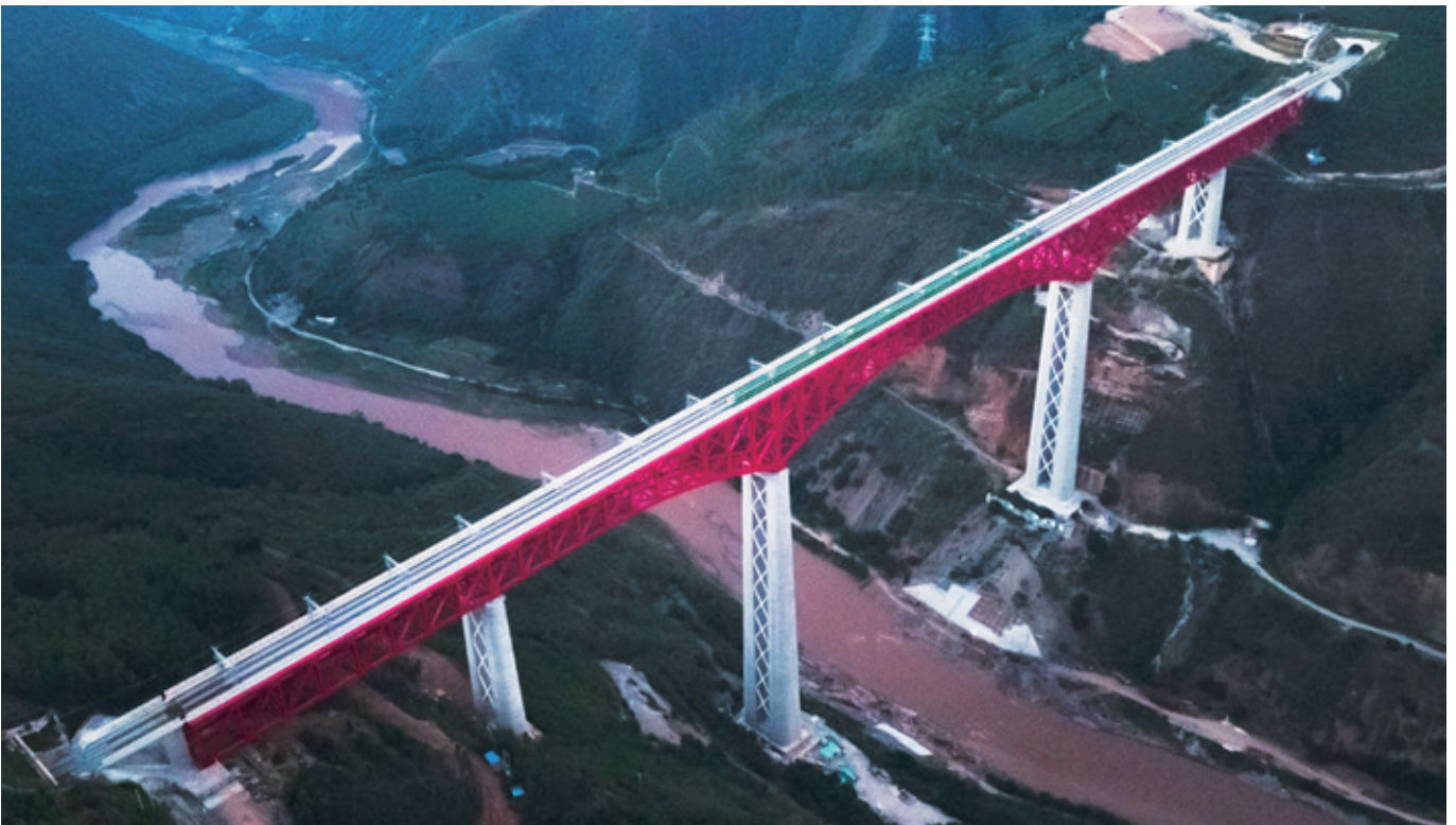
Aerial photo shows an electric multiple unit (EMU) train of the China-Laos Railway crossing a bridge over Yuanjiang River in southwest China's Yunnan Province, on December 3, 2021 (XINHUA)
