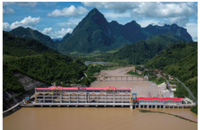
Aerial photo taken on July 13, 2022 shows the Nam Ou 1 hydropower plant of the Nam Ou River Cascade Hydropower Project in Luang Prabang, Laos (XINHUA)
